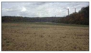
Photo 30 Crest of Subphases 1B and 1C. Temporary cover straw and seed at locations near grade. (Typical of Points 18,19, 21, 28, 29, and 30, Appendix A)
