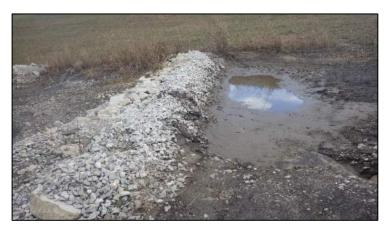
Photo 37 Looking southeast at check dam located on northwest side of Type I landfill. (Point 32, Appendix A)
