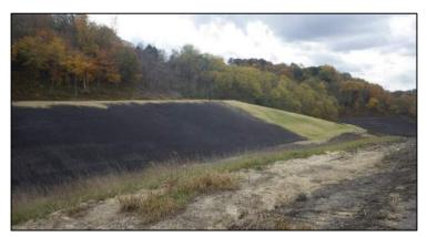
**Photo 29**Subphase 1D with boiler slag temporary cover (prior to waste placement), looking
