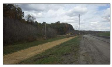
Newly constructed stormwater channel located on the north side of paved haul road. The ditch is not well defined in this area. (Point 36, Appendix A)
