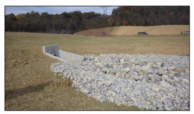
Photo 22 Looking northwest, downstream outlet headwall from the northeast sediment basin. (Point 11, Appendix A)
